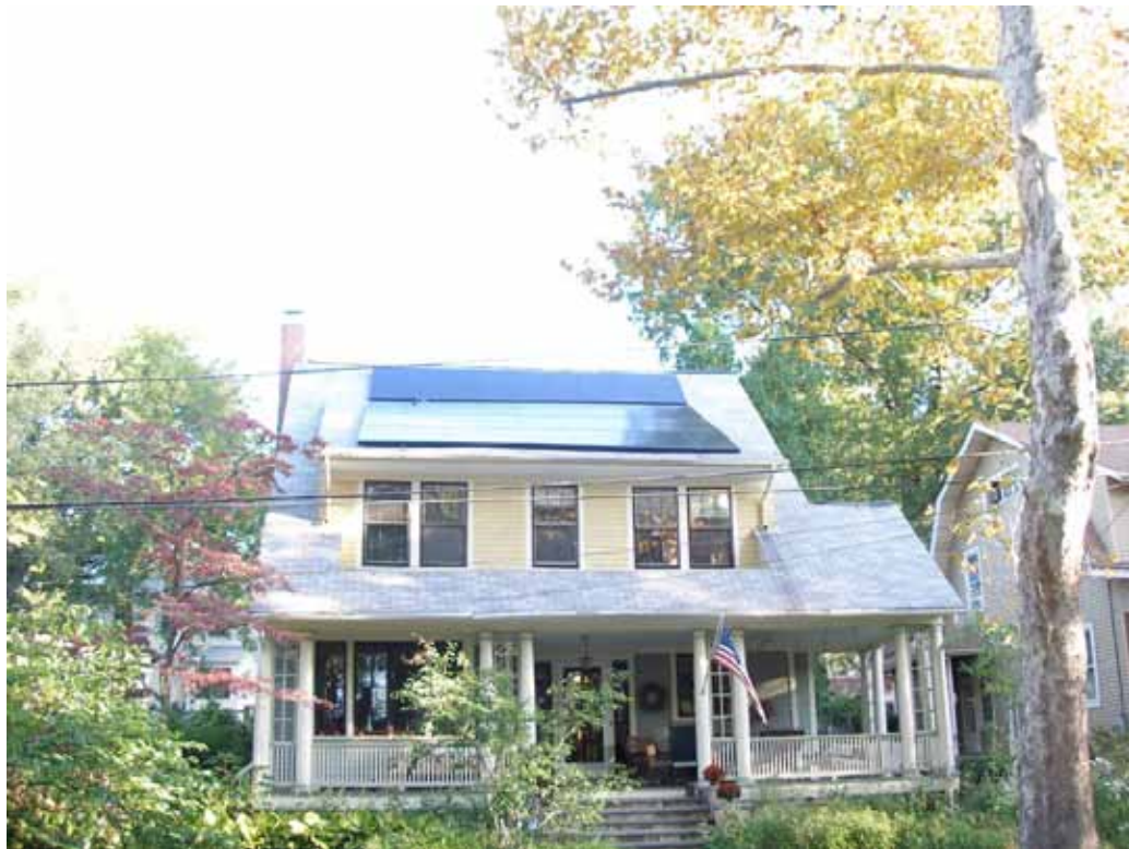
Figure 1: The Resch residence after additional installed capacity and SolarMagic. Notice that the new modules look identical to the old modules, and the SolarMagic units enabling this array are discreetly located below the modules. This new array has 7.4kWp of capacity.
